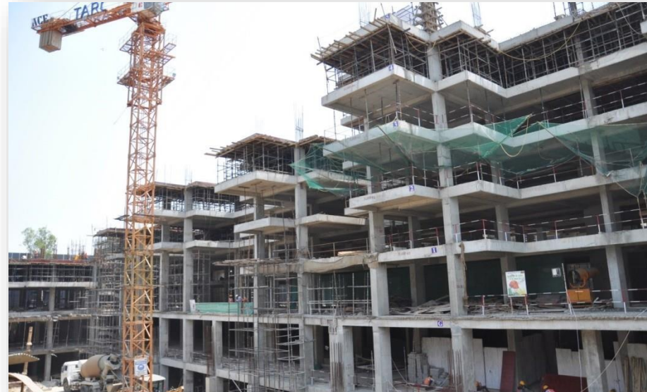
CURRENT SITE STATUS
